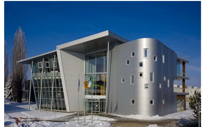
Kingspan Energy Centre in Hradec Kralove, Cz
