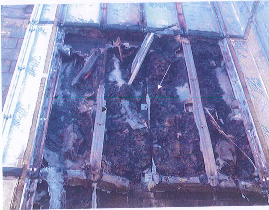
Burned Kooltherm K15 insulation and railings
