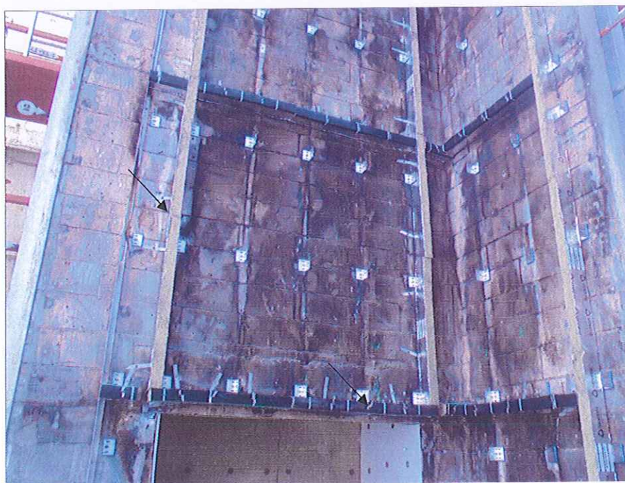
Vertical and Horizontal intumescent cavity barrier
