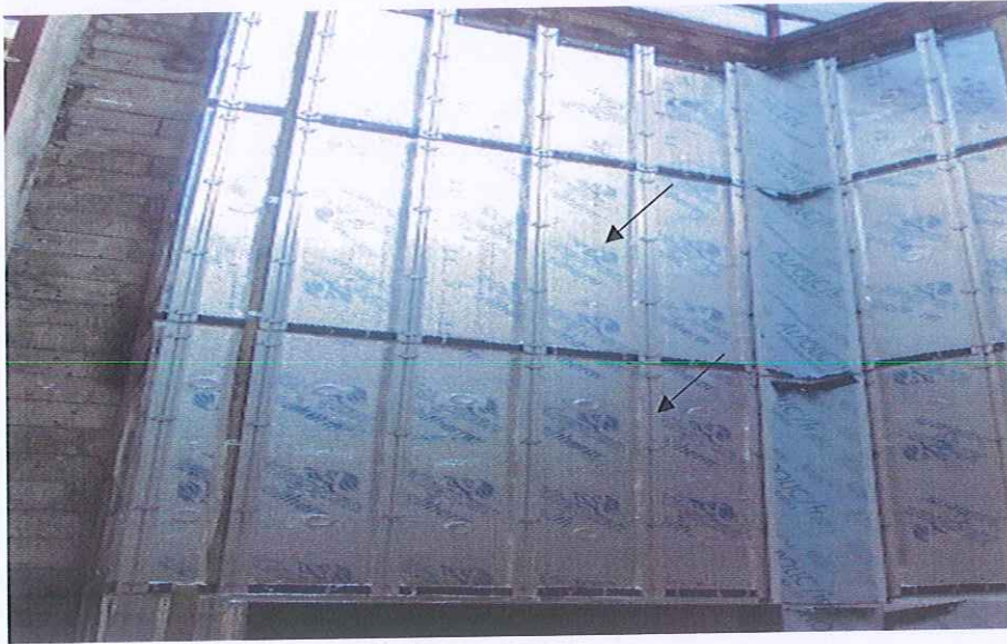
Kooltherm K15 Insulation and Railings
