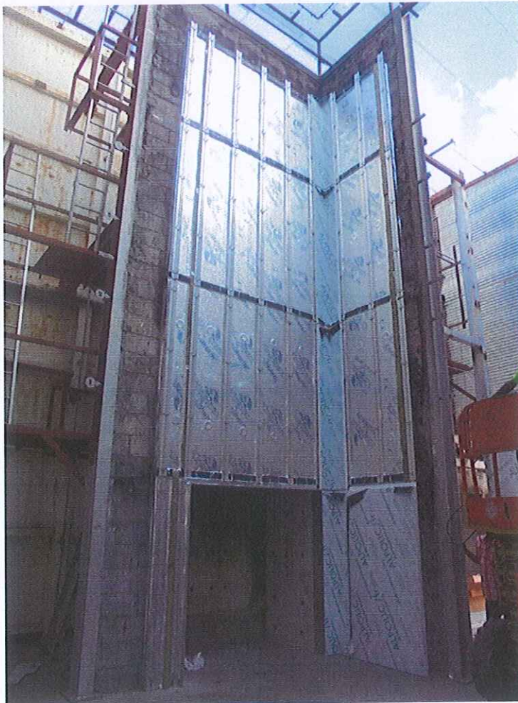
Cavity barrier and insulation
