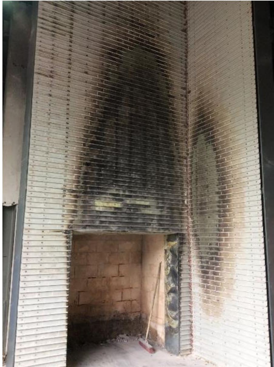
Figure 20. Damage to lower main and wing walls (Corium brick rail system).
