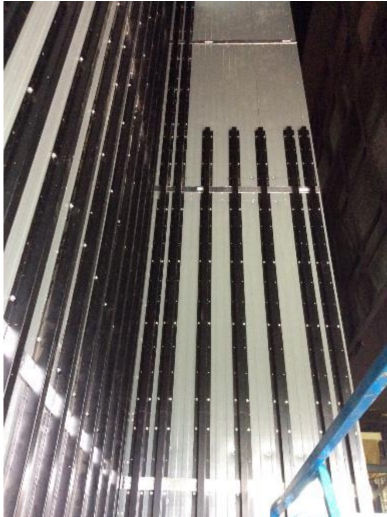
Figure 1. The system during construction showing top hat rails and fire breaks.
