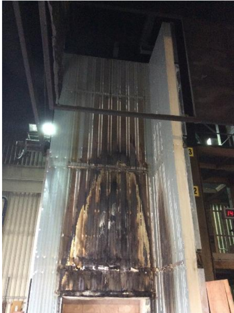
Figure 21. Damage to upper main wall (insulation layer).
