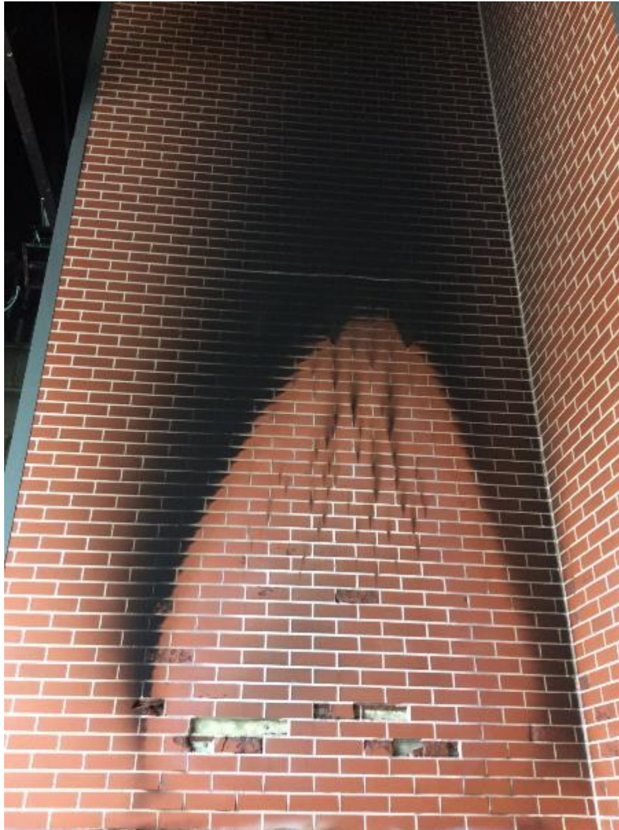
Figure 19. Damage to lower main wall (Corium bricks).
