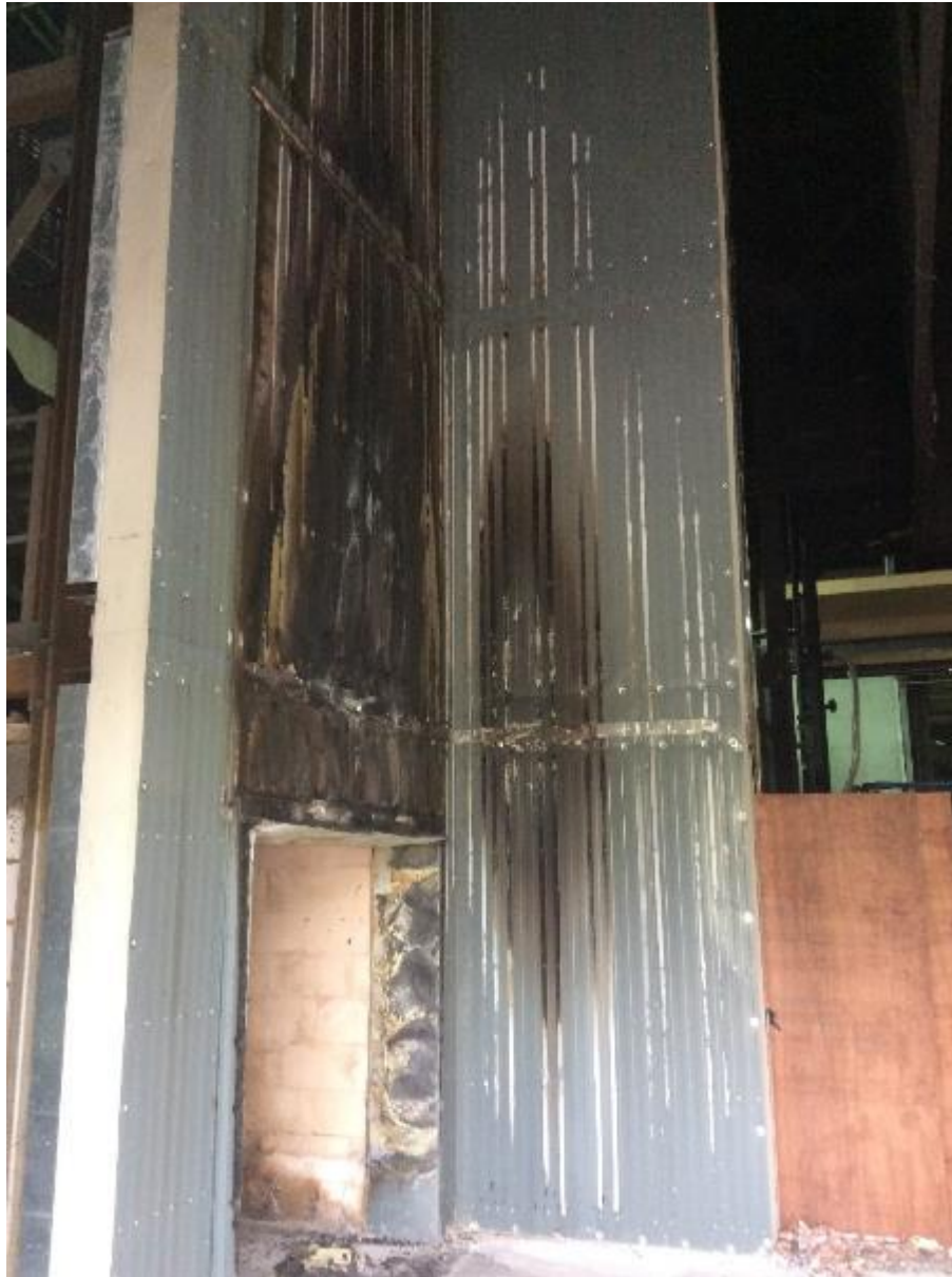
Figure 22. Damage to lower wing wall (insulation layer).
