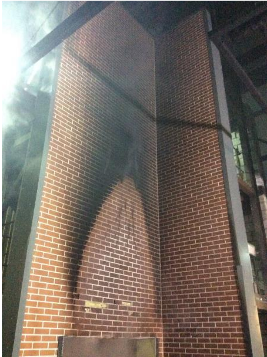
Figure 18. Damage to upper main wall (Corium bricks).
