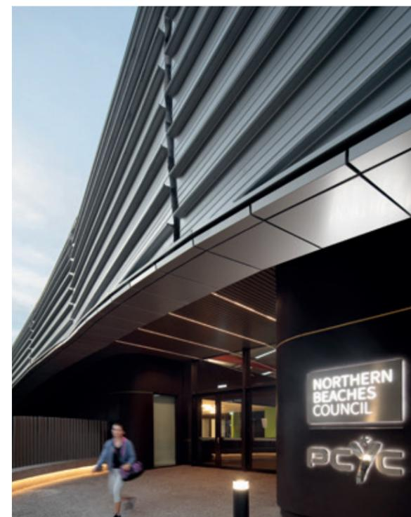
“One of the wonderful things about using KingZip is you can taper it, twist and bend it or curve it without losing the strength as a consequence. You can make irrational shapes very easily.”
