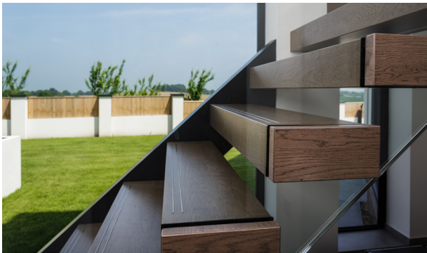
STAIRS Oak treads have been cut into the glass balustrade.
