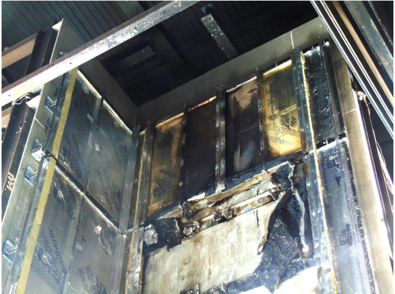
Figure 28. Damage to panels between a height of approximately 5000mm above the top of the combustion chamber and the top of the cladding system.
