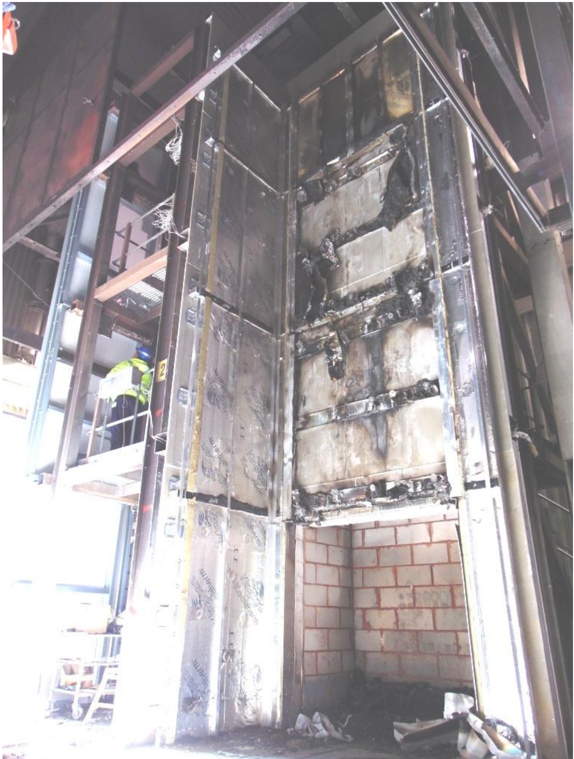
Figure 25. Full-height photograph of damage to insulation.
