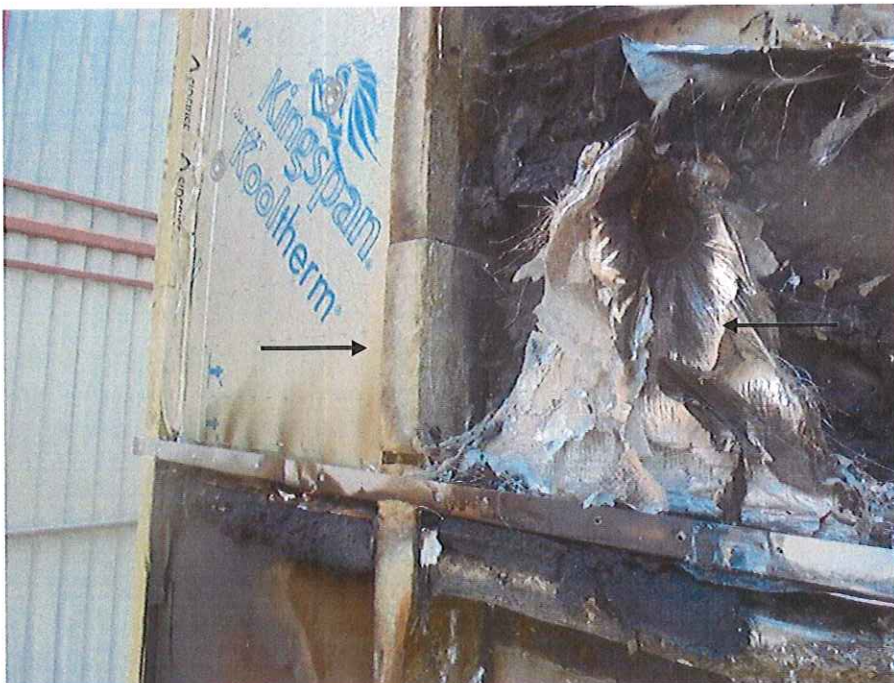
Vertical cavity barrier, insulation and railings on main wall
