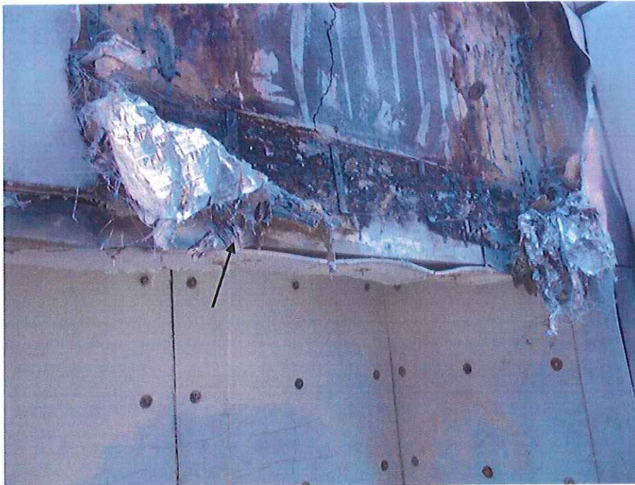
Cavity barrier above the combustion chamber
