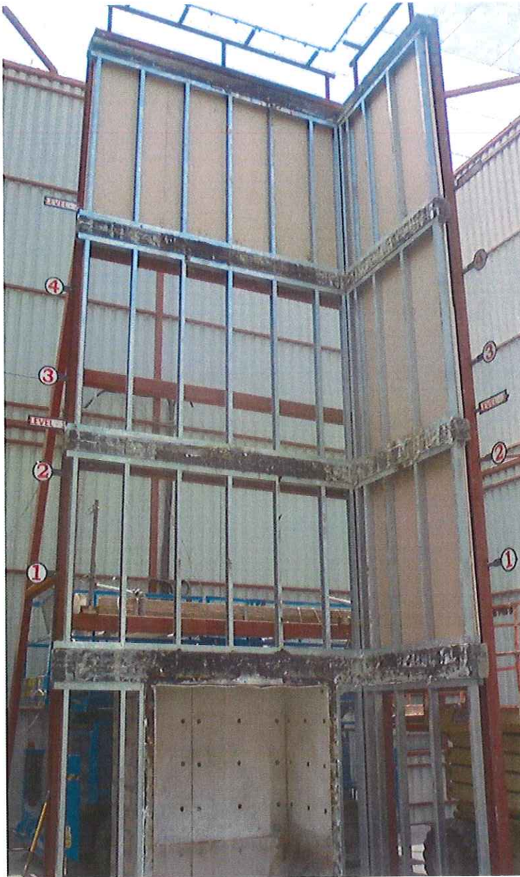
Kingframe SFS and plaster board
