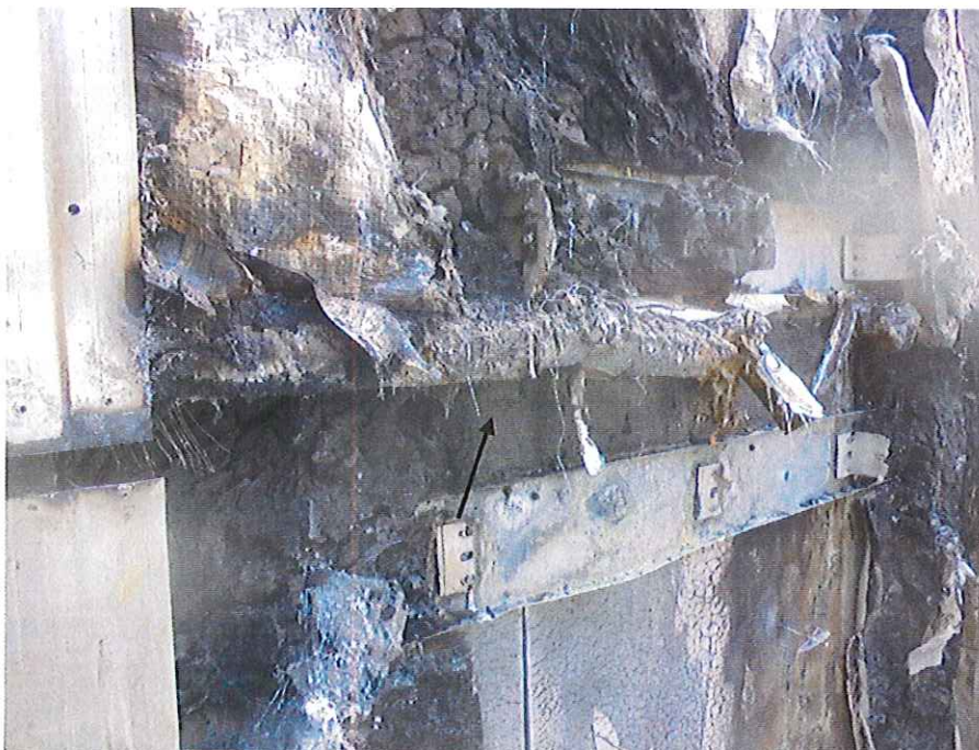
DLP C2753E/0016 Cavity barrier at level 1 main wall
