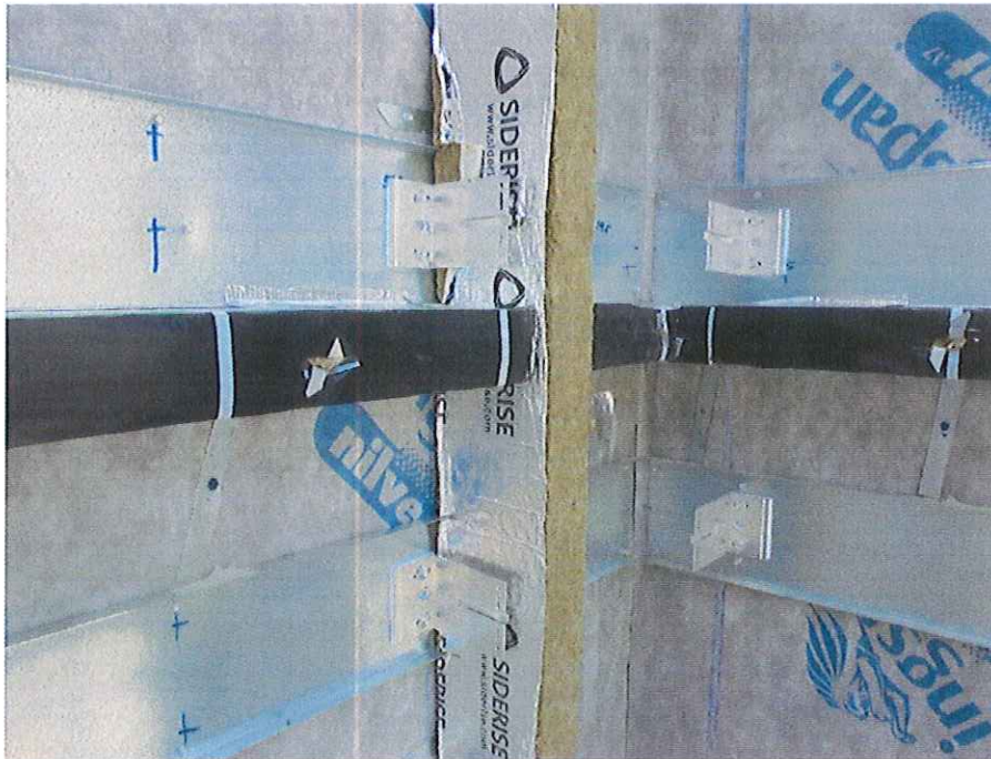
DLP C2753E/0324 Horizontal intumescent and vertical cavity barrier
