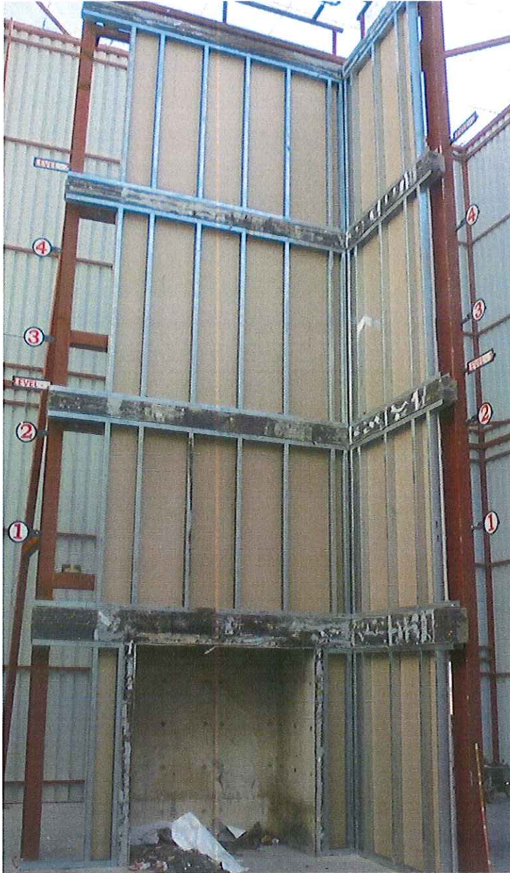
DLP C2753E/0015 SFS and plaster board
