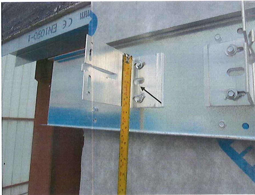
DLP C2753E/0297 Galvanized steel 'C' channel and Helping hand bracket
