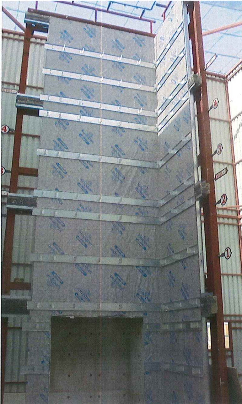
DLP C2753E/0291 Nilvent breather membrane, galvanized steel 'C' channel and Helping Hand bracket
