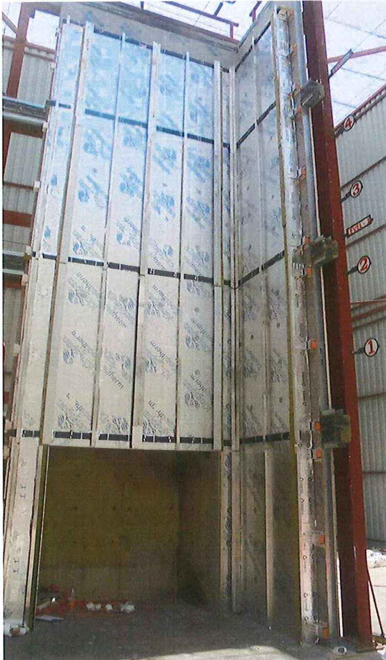
DLP C2753E/6571 Cavity barriers, Kingspan K15 insulation and carrier railings
