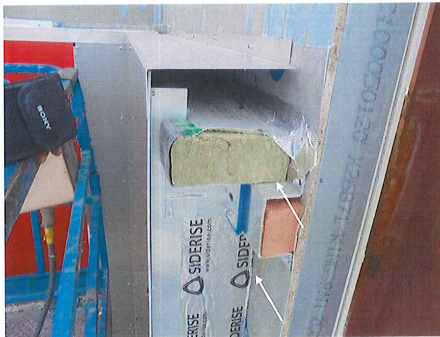
DLP C2753E/6165 Horizontal and vertical cavity barriers
