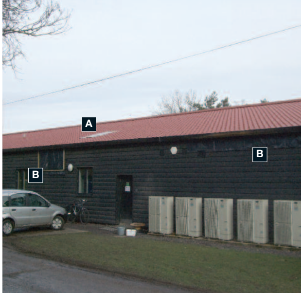
A: Vent cut in roof by fire service. B: Vents cut in wall by fire service.
