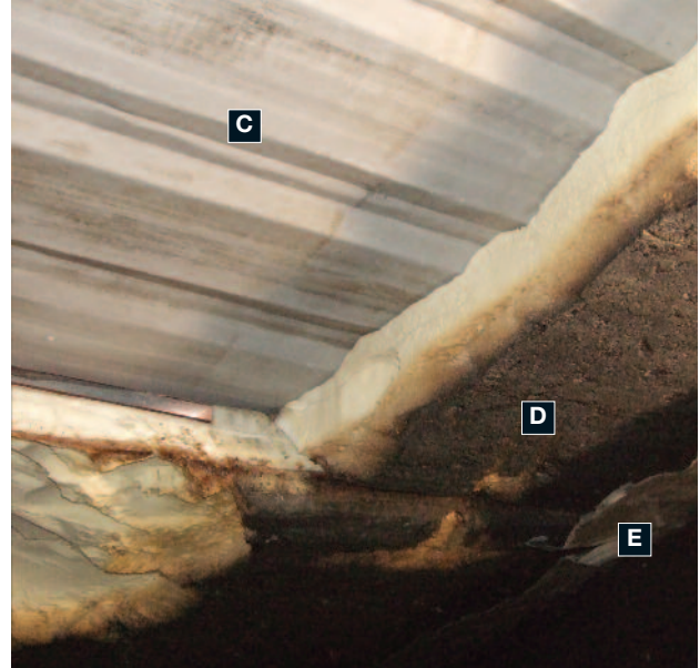
C: Temporary roof covering over hole in roof. D: PIR core showing delaminated lower surface and extent of through-thickness charring. E: Cut edge of lower steel skin of sandwich panel.
