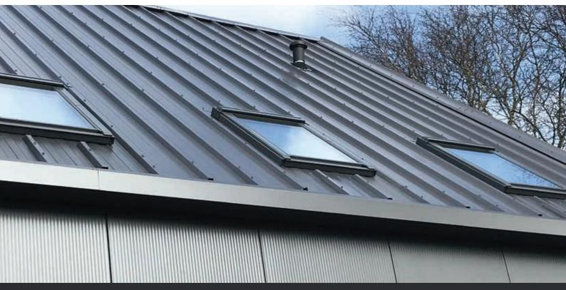
The high degree of pre-fabrication allows a short installation time
