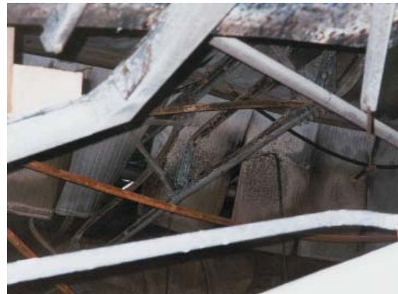
Boots, UK: Steel frame supporting polyurethane roof and wall panels. Severe fire resulting from ignition of flammable aerosol containers
