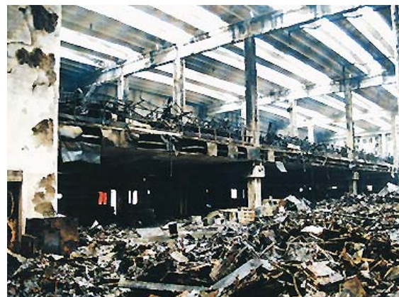
Fiege, Italy: Concrete frame - roof structure and metal clad wall. Structural failure leading to total building and contents loss
