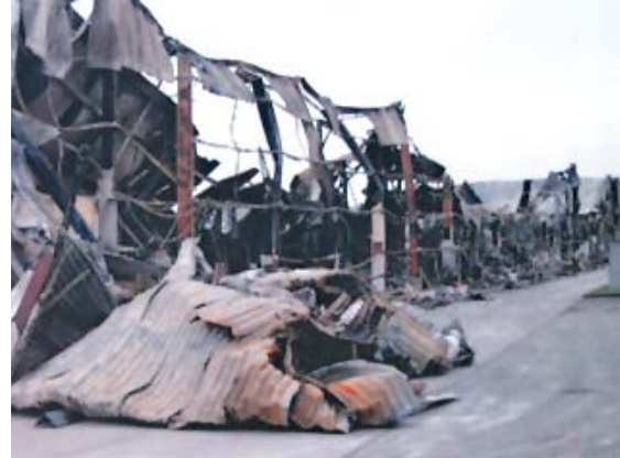
Panasonic, UK: Steel frame and site assembled mineral fibre roof and wall system. Structural failure leading to total building and contents loss.
