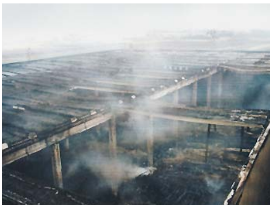
Fiege, Italy: Concrete frame - roof structure and metal clad wall. Structural failure leading to total building and contents loss
