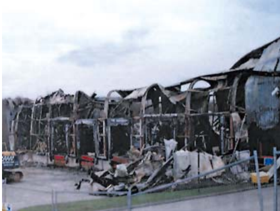
Panasonic, UK: Steel frame and site assembled mineral fibre roof and wall system. Structural failure leading to total building and contents loss.
