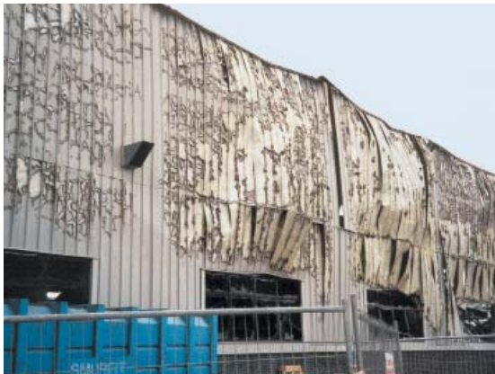
Boots, UK: Steel frame supporting polyurethane roof and wall panels. Severe fire resulting from ignition of flammable aerosol containers
