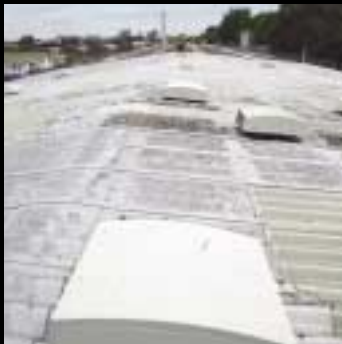
With the removal of asbestos roofing sheets, the KS1000 RW Trapezoidal in Goosewing Grey refurbishment program was applied along with roof lights
