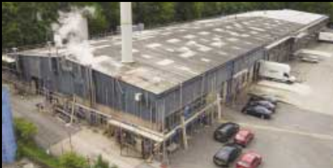
With the removal of asbestos roofing sheets, the KS1000 RW Trapezoidal in Goosewing Grey refurbishment program was applied along with roof lights
