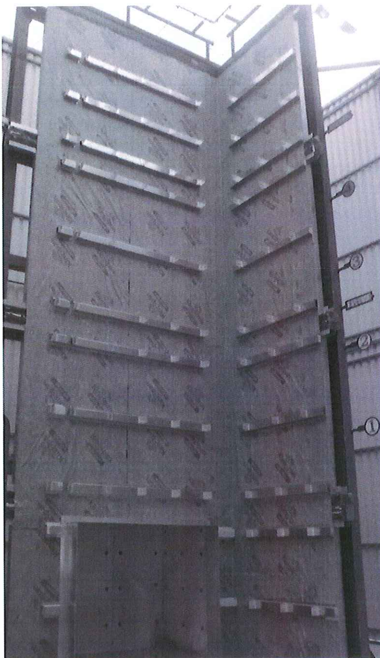
DLP C2753I/2008 Nilvent breather membrane, Top hat and Helping hand brackets
