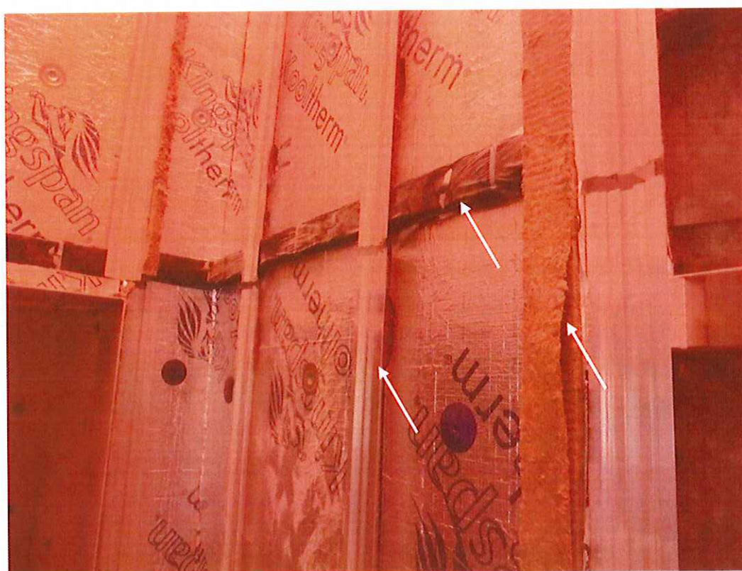
DLP C2753I/2051 Cavity barriers, railings and Kooltherm K15 insulation
