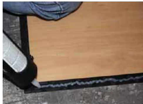
Seam sealer for waterproof installation
