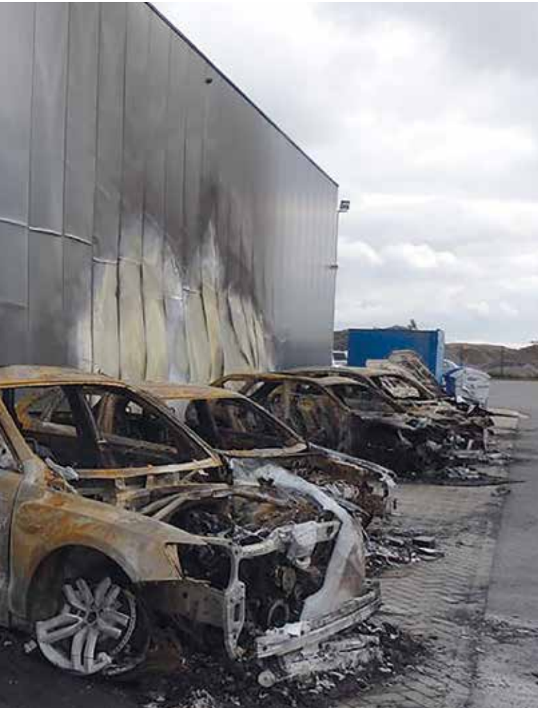
No evidence of fire penetration to interior of the workshop
