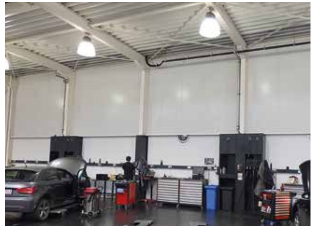
No evidence of fire penetration to interior of the workshop
