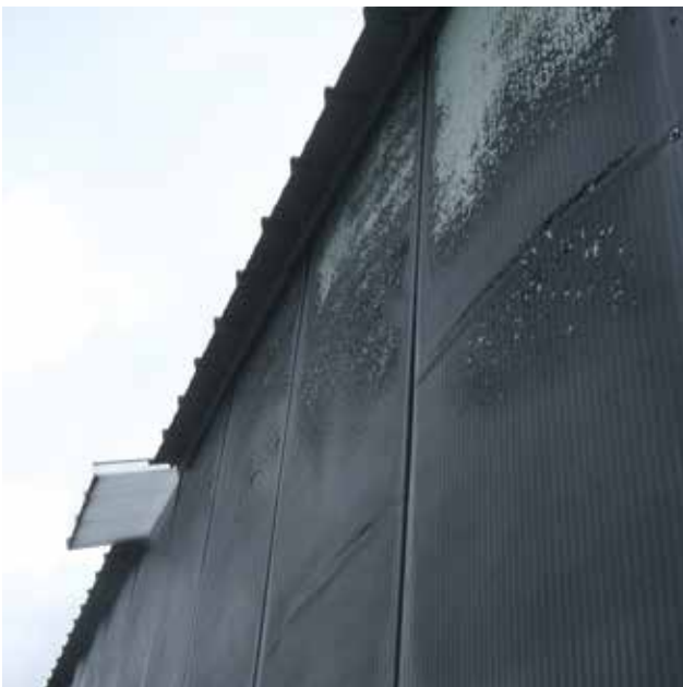
Close-up of damage to the Kingspan ECOsafe PIR wall cladding of building A.
