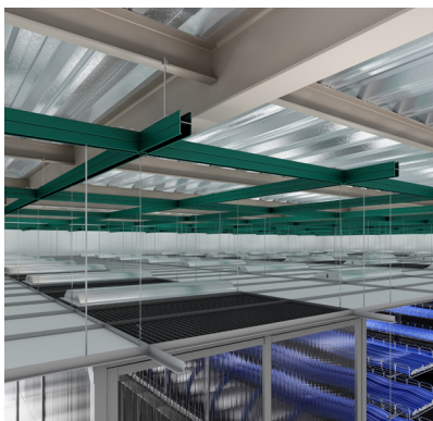
Traditional ceilings require an interstitial strut grid for hanging heavy items.
