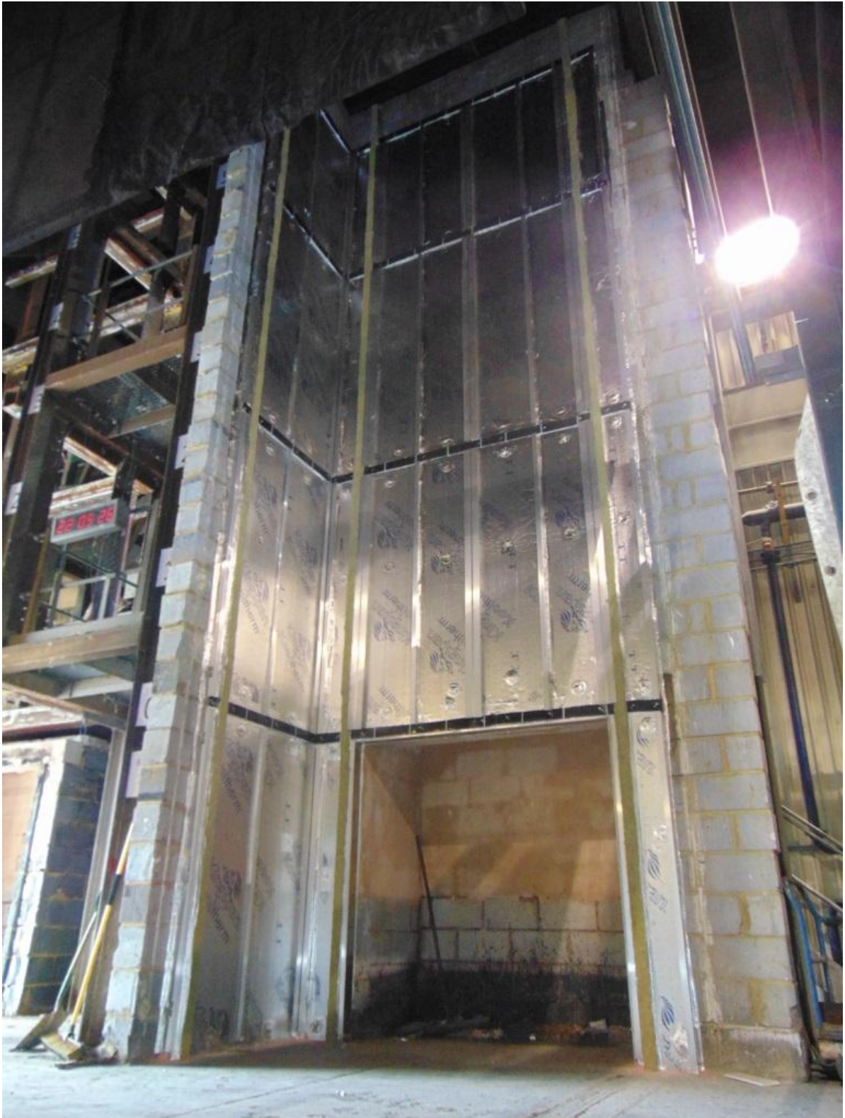
Figure 6. Installation of 'L'-shaped rails.
