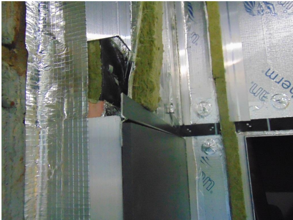
Figure 8. Horizontal panel joint flashing.
