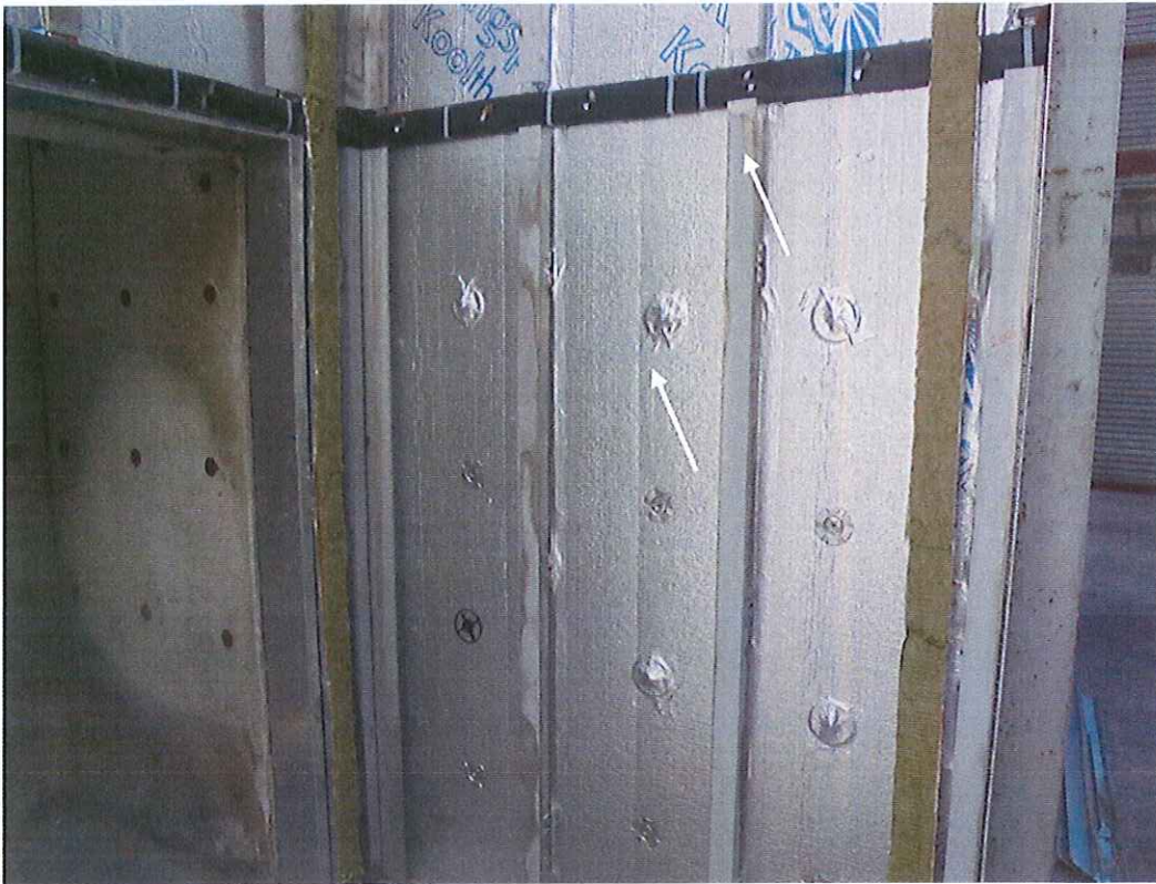
Photo 5 Kingspan Kooltherm K15 insulation and railings
