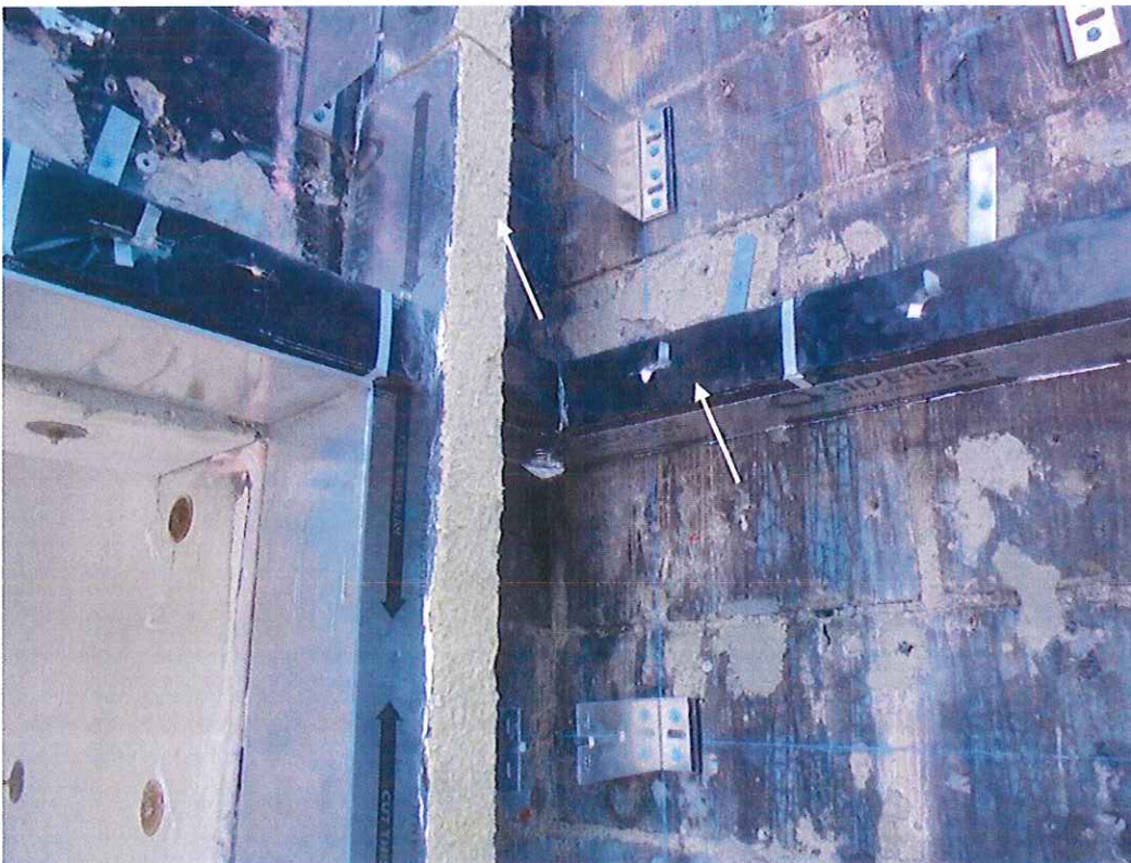
Photo 4 Vertical and horizontal intumescent cavity barriers
