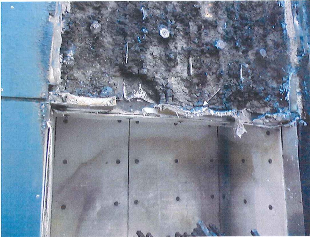
Photo 19 Cavity barrier at the top of combustion chamber
