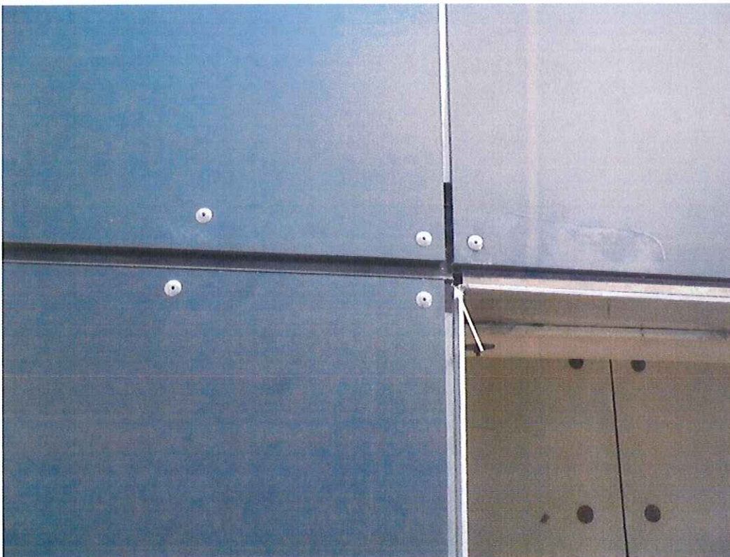
Photo 6 Trespa Meteon FR panel fixing and aluminium bird peak profile
