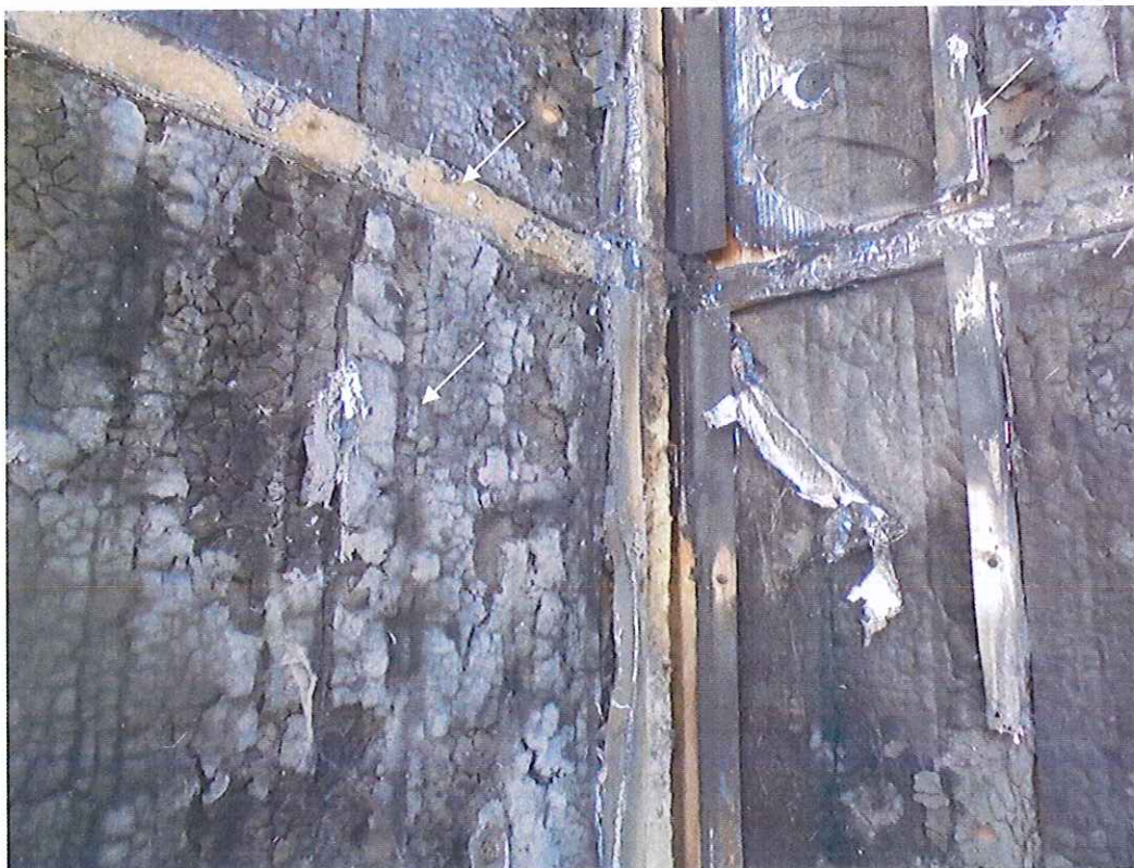
Photo 20 Cavity barrier, Kingspan Kooltherm K15 insulation and railings at level 1
