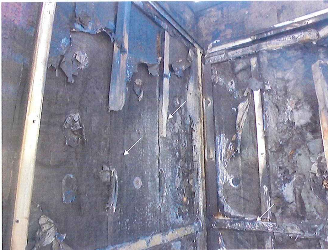
Photo 21 Cavity barrier, Kingspan Kooltherm K15 insulation and railings at level 2
