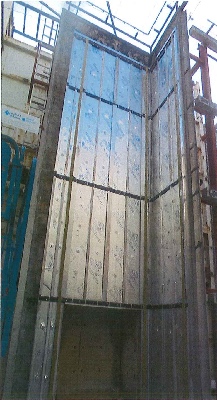
Photo 2 Cavity barriers, Kingspan Kooltherm K15 insulation and railings
