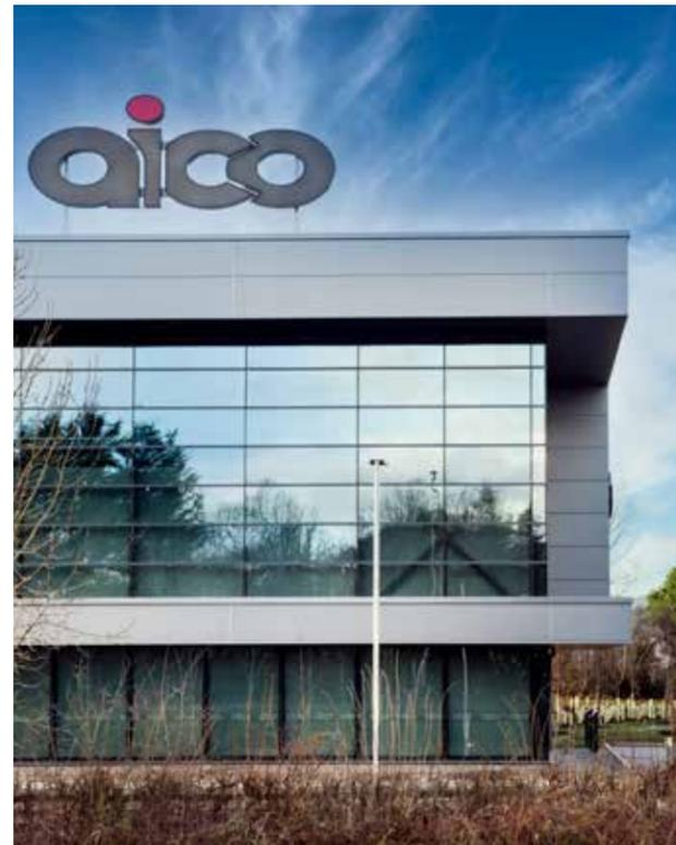
"Due to the building containing such a large glazed frontage, we needed to achieve a significant gain in the thermal performance of the rest of the building envelope. By specifying Kingspan insulated roof and wall panels, we were able to achieve this whilst still maintaining the desired aesthetic."
