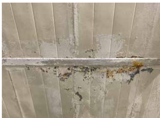
Corrosion damage on ceiling panels caused by inadequate coating selection.
