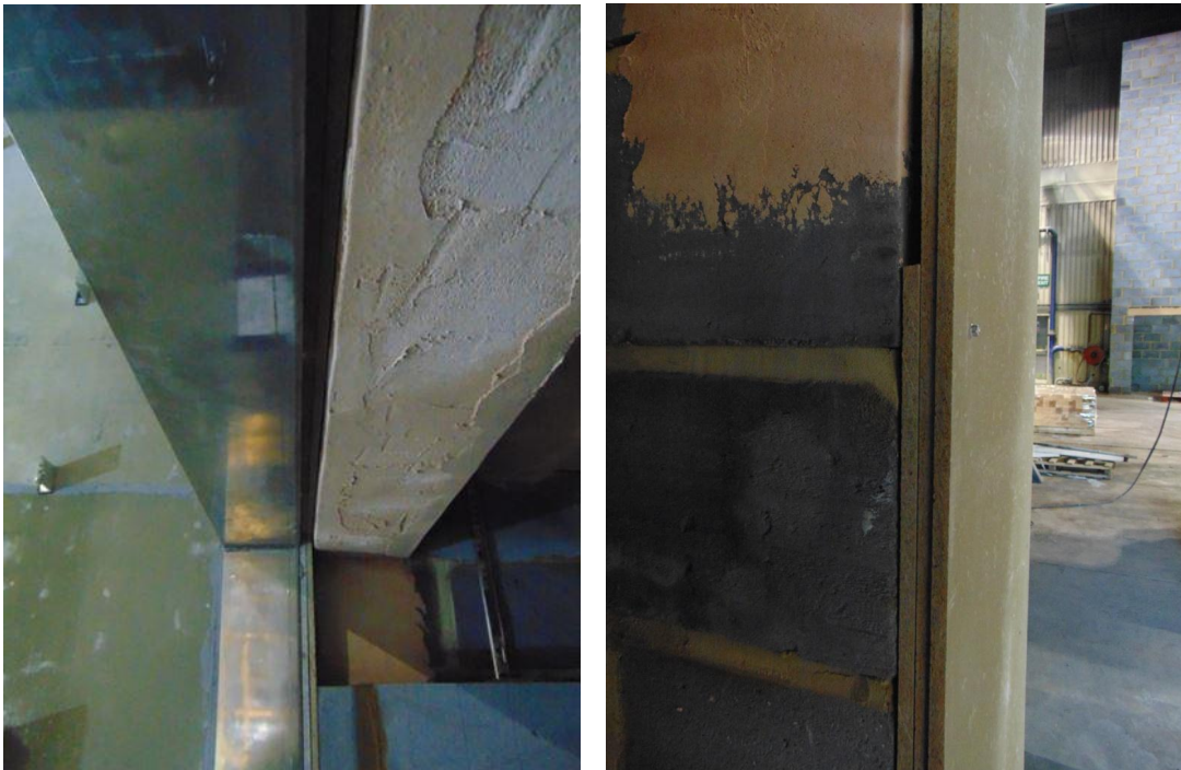
Figure 8. Double (left & top)/triple (right) layer of cement board around combustion chamber opening.
