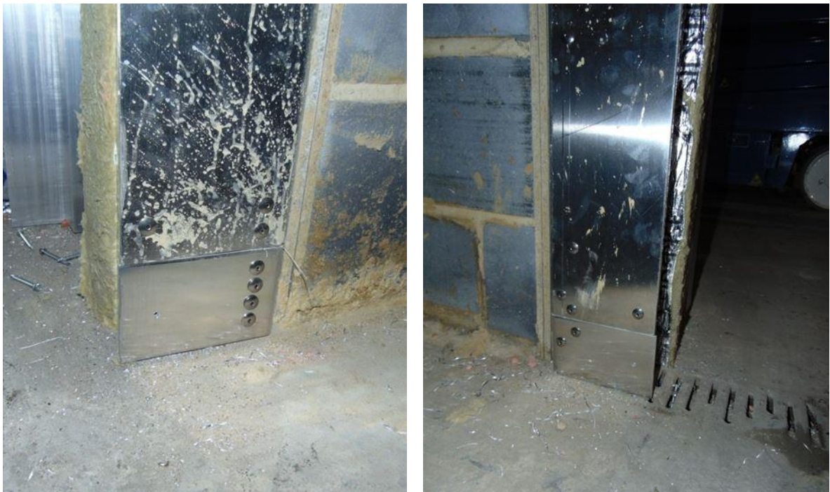
Figure 13. Additions to combustion chamber surround pod base.
