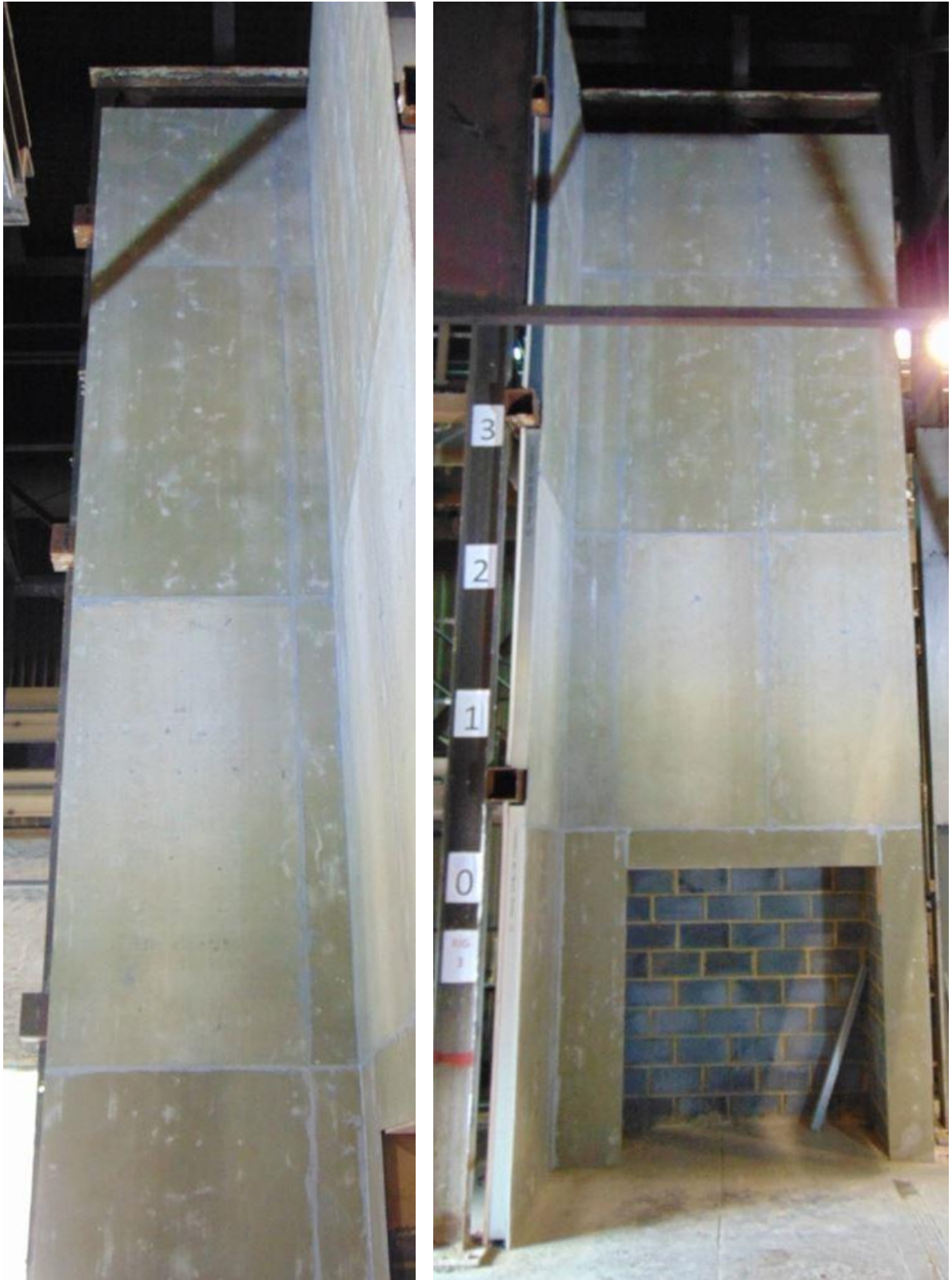
Figure 5. Installation of cement bonded particle board.
