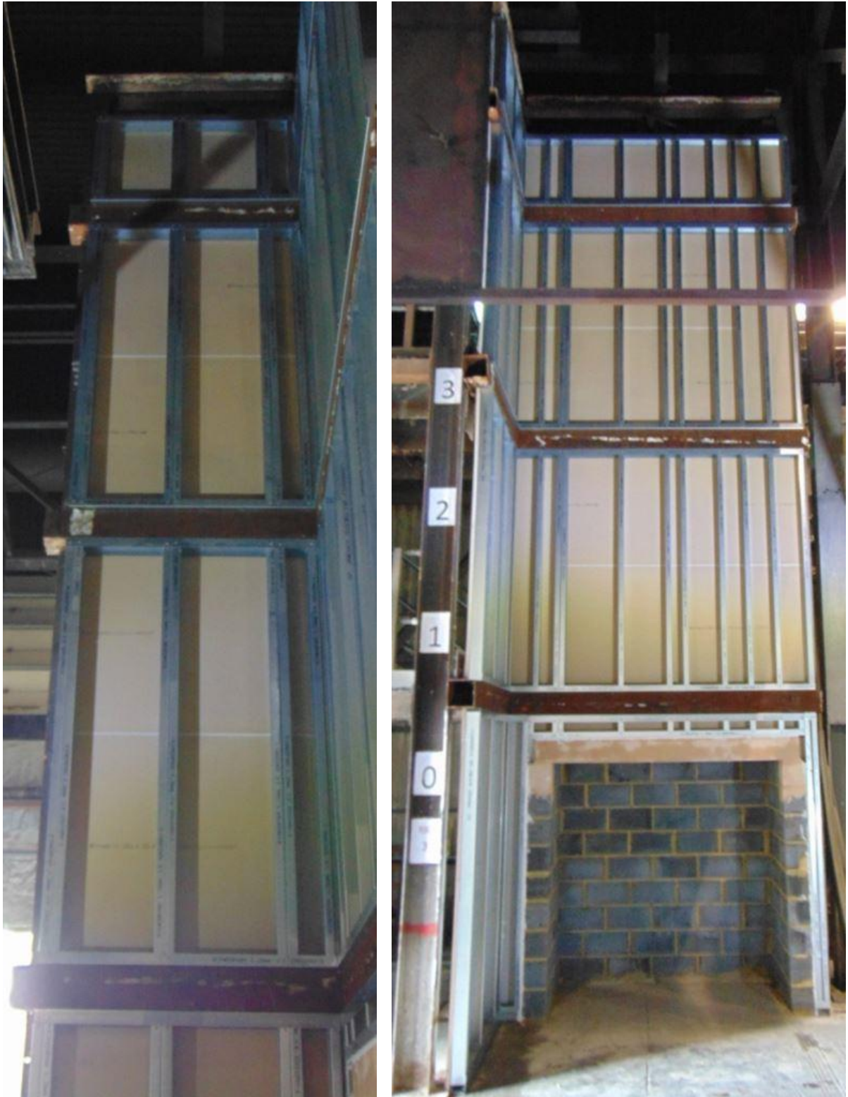
Figure 3. Installation of SFS and plasterboard.
