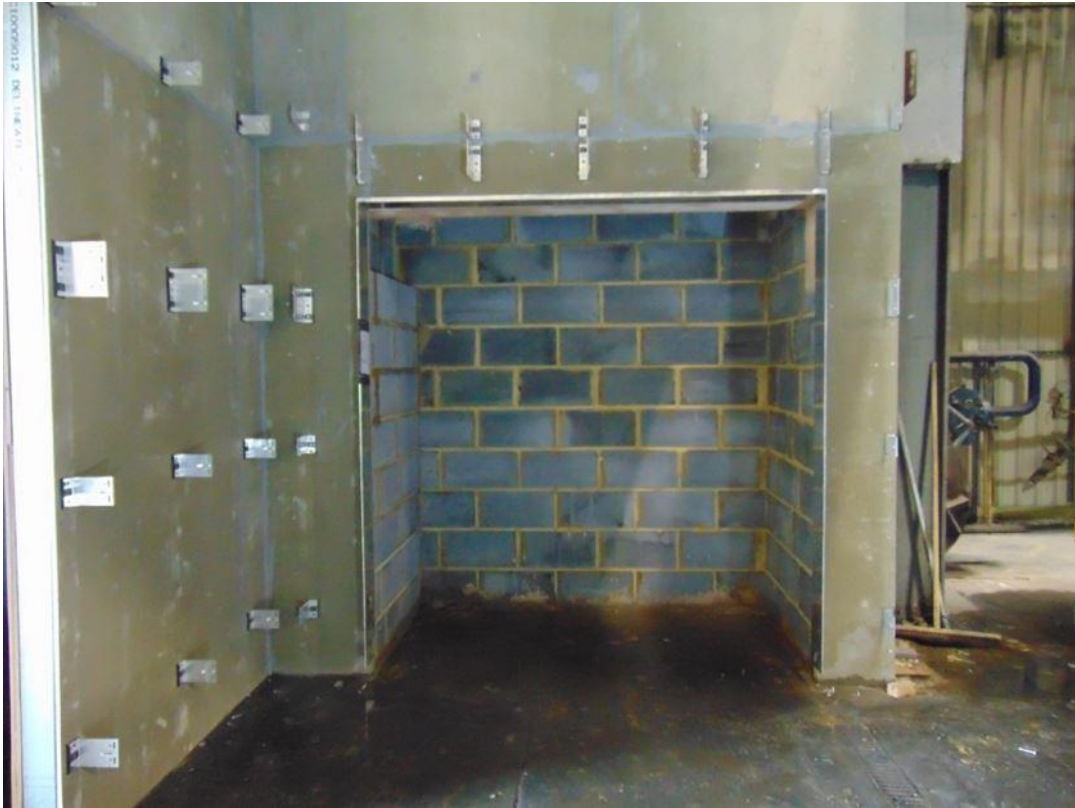
Figure 7. Installation of combustion chamber surround pod.
