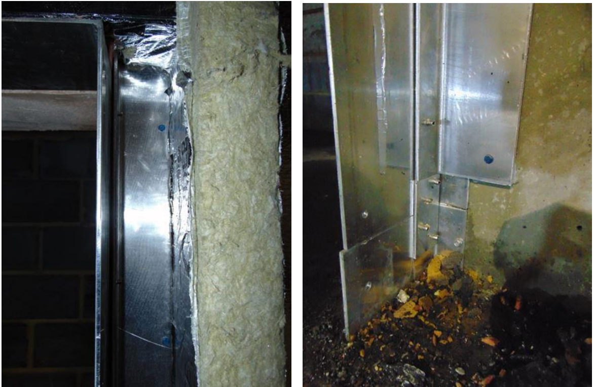
Figure 12. Additions to combustion chamber surround pod.
