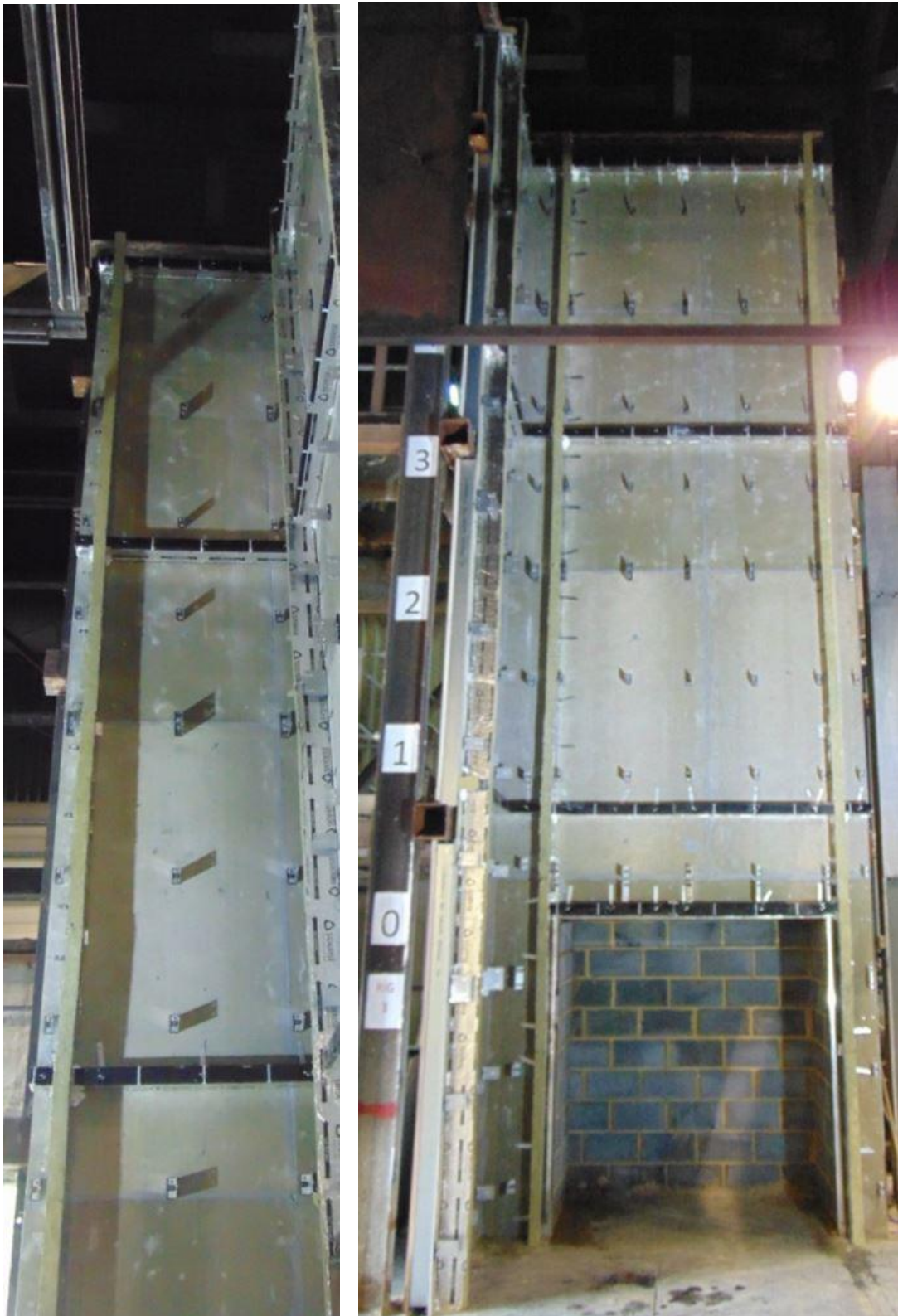
Figure 9. Installation of vertical and horizontal cavity barriers and aluminium brackets.
