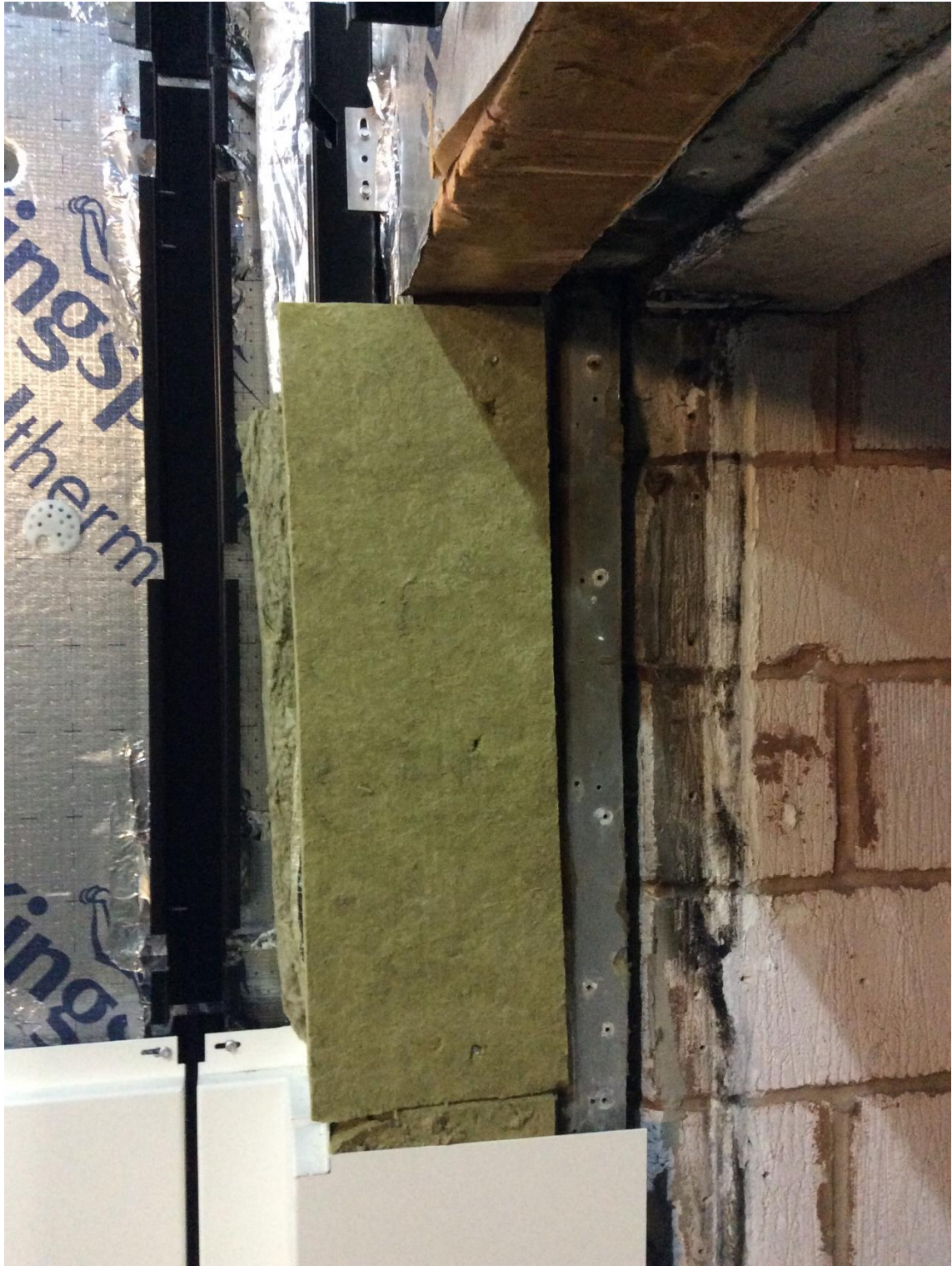
Figure 5. Combustion chamber surround detail.
