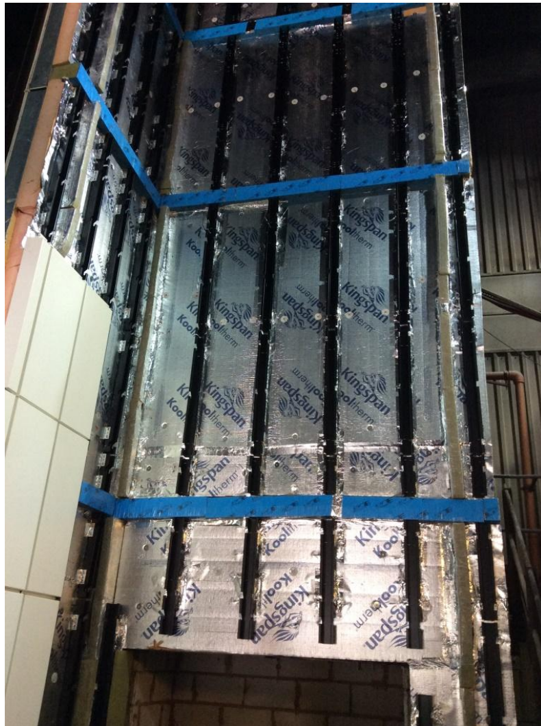
Figure 3. Installation of insulation, cavity barriers and panels to wing wall.
