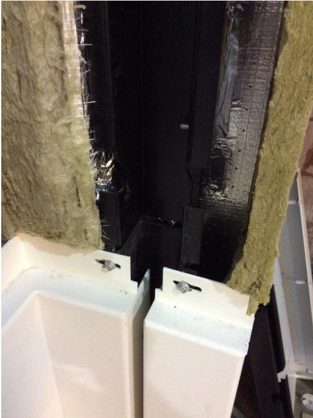
Figure 4. Panel fixing detail.
