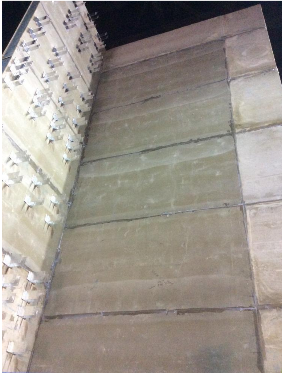
Figure 1. Installation of sheathing board and wing wall brackets
