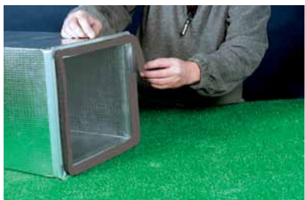
Figure 10.5 Affixing Self-Adhesive Gasket
