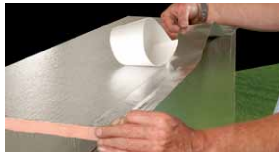
Figure 2.10 The Taping Procedure
