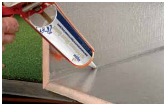
Figure 2.11 The Sealing Procedure
