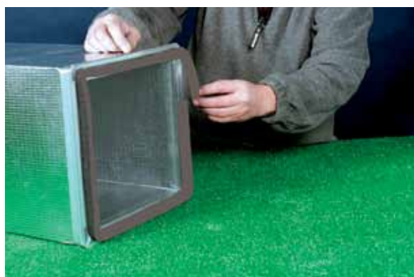
Figure 10.5 Affixing Self-Adhesive Gasket
