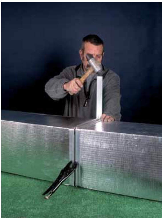
Figure 10.6 Fitting Bayonet Cleats
