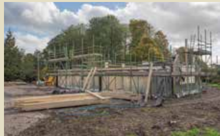
Once the site was prepared, the timber frame was delivered and quickly erected
